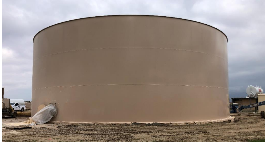
Figure 1-2: Newly-Installed Storage Tank
